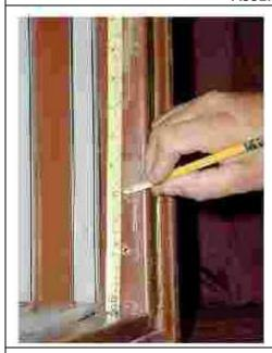
Do a Window Bar Lay Out on paper. Take Guidance from the lay out example shown above. Once you have lay out ready Transfer/ Mark measurement to Window Frame. This will help you to determine where the first horizontal bar needs to install
